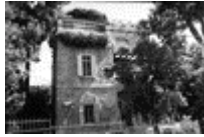
18 A former Arab house at Hovevei Tzion St. Jerusalem, the Middle East, June 28, 2001
