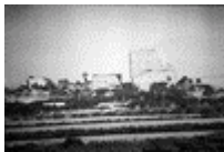
15 View of Crusaders Castle (now a military camp) in Atlit (south from Haifa) from a train. The Middle East, April 19, 2001
