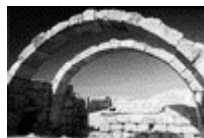
15 Remains of a Roman house with arches. Avdat, the Middle East, February 15, 2001
