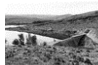
31 A dam of a polluted water reservoir. Yeroham, the Middle East, March 8, 2001
