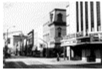
33 Main St. in downtown Lafayette. Indiana, January 18, 1998.
