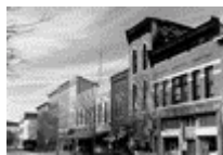
24 Main St. in downtown Lafayette. Indiana, January 18, 1998.
