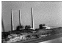
18 Smoke pipes of Hadera power station. The Middle East, April 22, 2000
