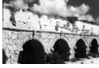
24 Roman aqueduct in Caesaria. The Middle East, April 22, 2000
