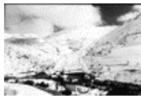
03 Cableway to Mt. Hermon in Golan Heights. The Middle East. February 19, 2000
