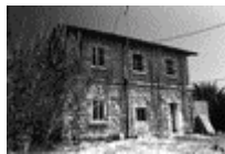
24 Home of the manager of Turkish Railway Station. Beer-Sheva, the Middle East, April 24, 2000
