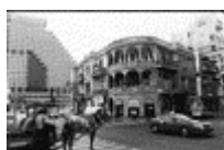
01 A hotel at intersection of Trumpeldor and Hayarkon St. Tel Aviv, the Middle East, November 23, 2000
