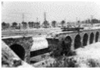
06 Railroad Turkish Bridge (blown up by Israelis in 1948 for security). Beer-Sheva, the Middle East, April 13, 2000
