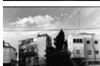
10 Houses at Gruzenberg St. Tel Aviv, the Middle East, November 23, 2000
